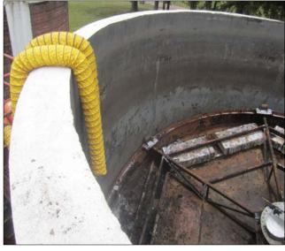
The cement digesters were built in the 1930's and play a key role in the breakdown of sanitary waste before it reaches the primary and secondary treatment systems. After partially disassembling one digester, it was discovered the structures were in remarkably good condition for their age.
