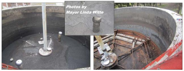
The Public Works Department recently discovered some problems within the city's three sewer treatment plant digesters and is working on an interim remedy for the situation.
