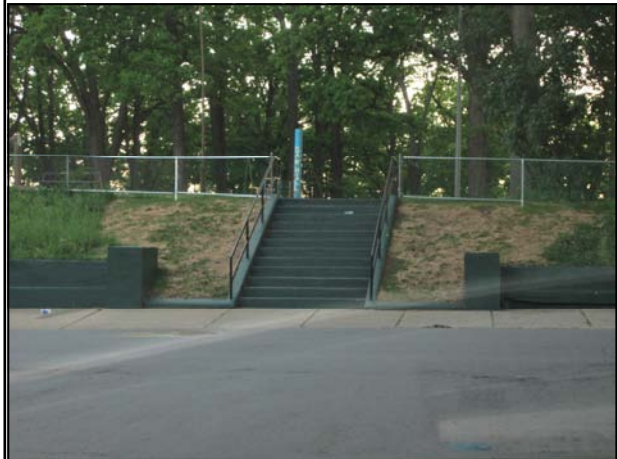
The staircase leading from Laurens Street to Oak Hill Park has been repaired by contractors and the bank has been re-seeded. Other work is under way at Oak Hill Park for public enjoyment!
