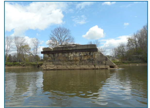
Pier from old railroad bridge in Allegheny River, Allegany
