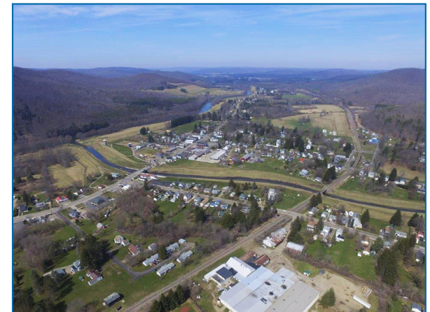
View of Portville's flood levees from above, with the Allegheny River on the left and Dodge Creek running through the middle
