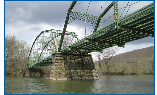
Vandalia Bridge at Nine Mile Road, Allegany
