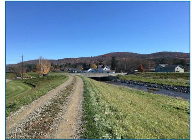
View east along flood levee to the North Main Street Bridge with Dodge Creek on the right
