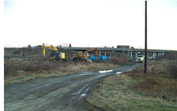
VIEW OF ONGOING SITE REMEDIATION
