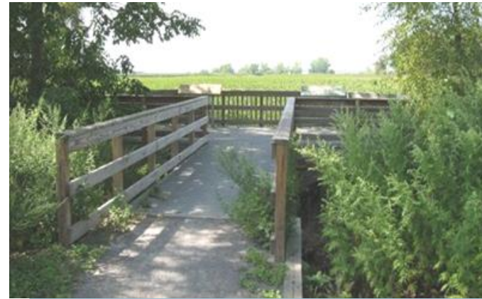
WETLAND OVERLOOK WITH INTERPRETIVE PANELS AT TIMES BEACH IN BUFFALO, NY.
