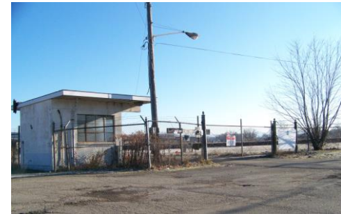
FORMER GUARD POST AND PROPERTY ENTRANCE
