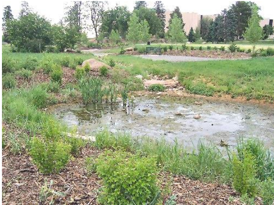
AN EXAMPLE OF A STORMWATER RETENTION AREA DEVELOPED AS A WETLAND.
