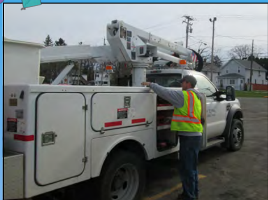
Left: City Electrician Dustin Kelley at War Vets Park installing lighting near the tunnel to Bradner Stadium.
