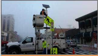
Olean's North Union Street said good-bye to its final traffic signals in the summer. To aid street crossing for pedestrians new devices were installed at a number of the crosswalks. The devices are activated by a hand motion. The device will say, "Lights are flashing." The flashing lights give motorists the heads up that there are pedestrians about the cross the street—and allows for a safe crossing for Olean's pedestrians.
